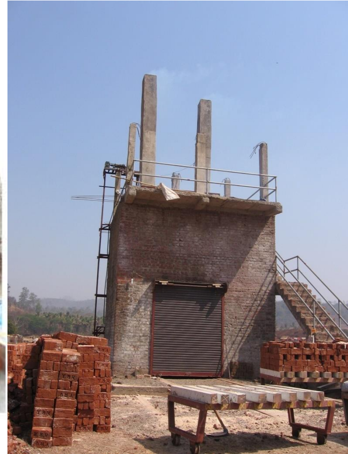
Vertical Shaft Brick Kiln
