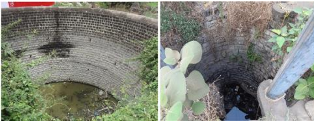
Assessing the drinking water access Chikurde, Maharashtra
