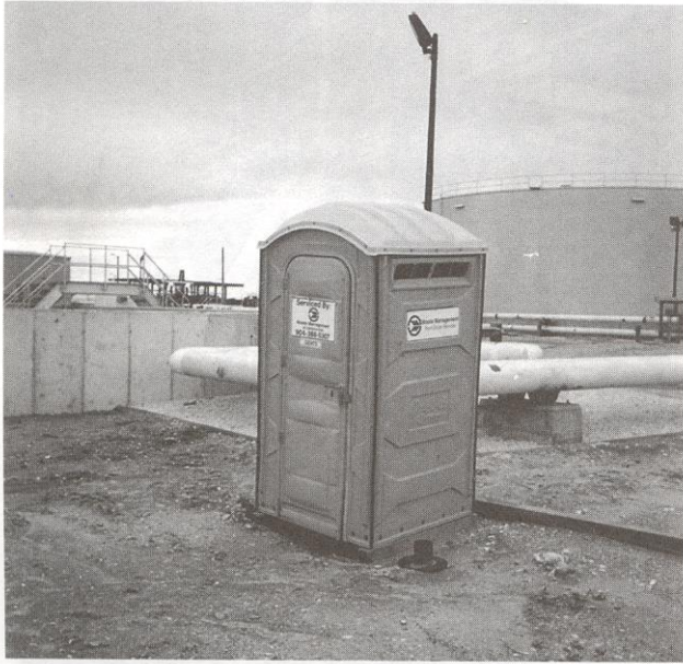
Portable toilet at job site
